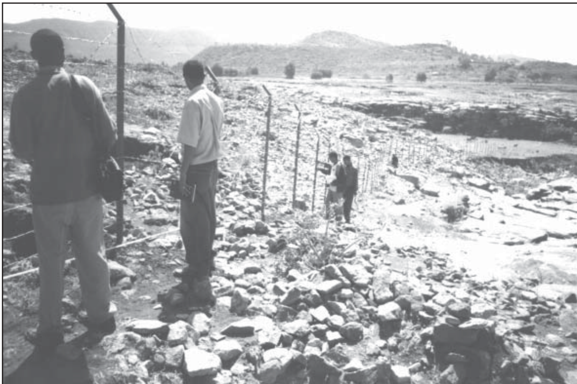
Figure 4. Permanent fencing at Mai Adrasha.
